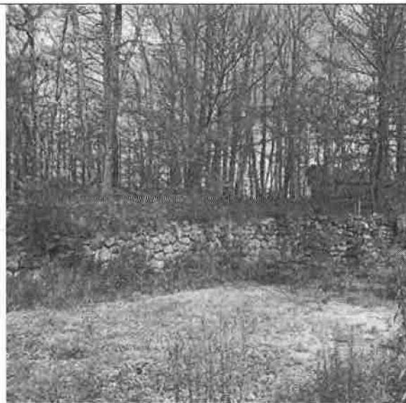
Figure 19 stone retaining wall near gravel/sandy area
