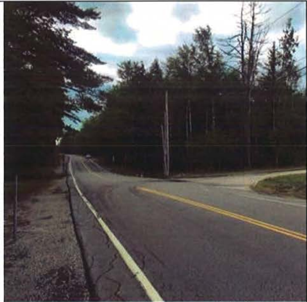
Figure 44 NH Route 153 south, NHDOT Patrol shed xx entrance visible on right
