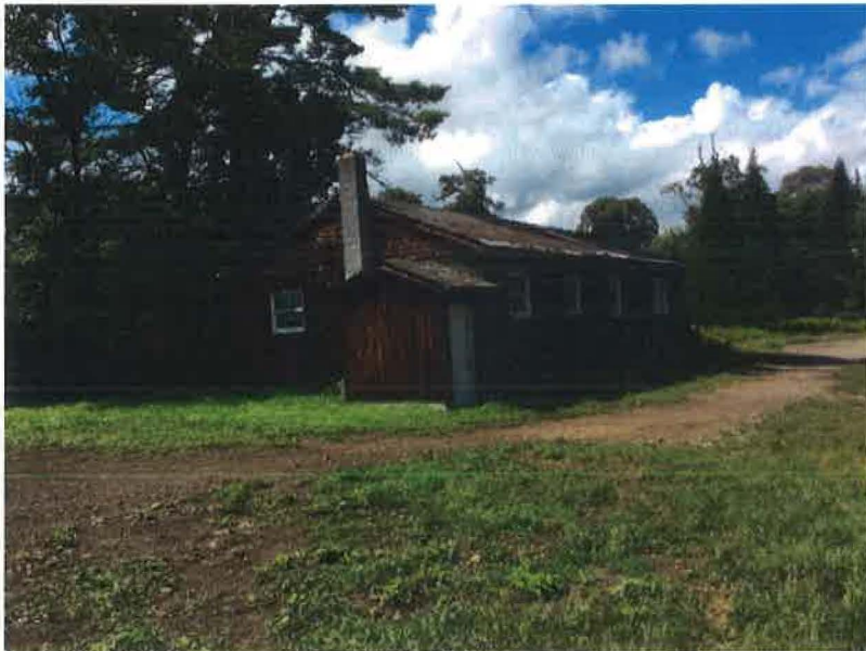
Looking west of the single-story home.
