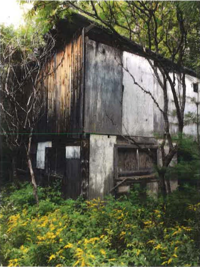
Looking east in parcel at the detached ancillary building.
